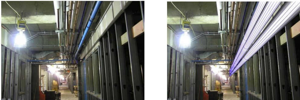
Figure 2 Augmentation of a real scene (left image) with a virtual overlay (right image). The appropriate placement of the virtual object was determined by the identification and positioning component.
